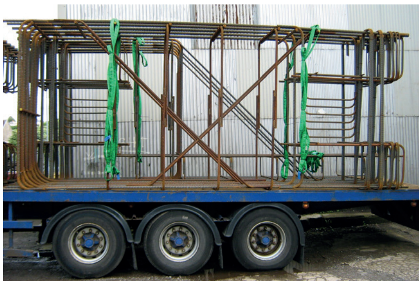
Two cages positioned end-to-end on a trailer. The top bars are spaced 50mm apart at 235mm centres, and the largest cage weighed 5.1 tonnes.
